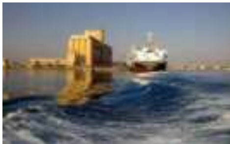
Port Sudan silo
